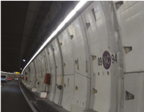
Illustration 29 – Alphanumeric Code for M30-Bypass. In this case, the same code is placed also on the walls of the emergency gallery that is below the traffic space.
