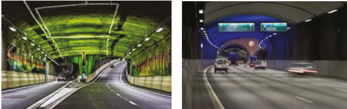
Illustrations 27 & 28 – design and signage of an exit on the Southern Link in Stockholm
